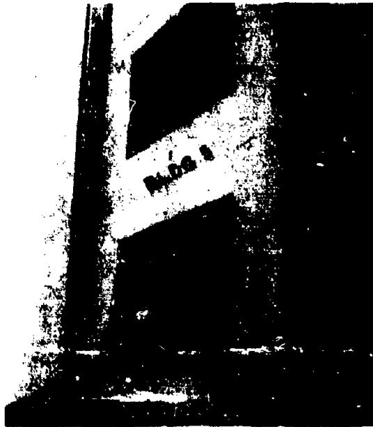
Figure 4.42 Post-Walnut, (Item 26) Station 3.1.1, close-up of Building 5, a reinforced-concrete frame structure. Pressure level: Walnut, 16 psi.
